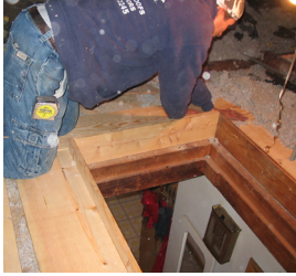
CEDA contractor installs an attic hatch before insulating.
